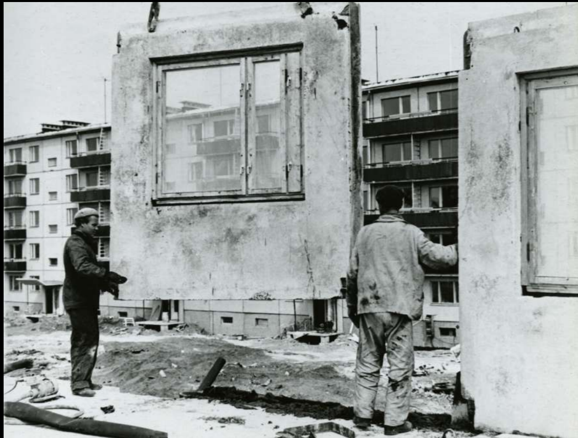
Mustamäe housing district, Tallinn, Estonia. Window panel. Architects Voldemar Toppel, Toivo Kallas, Lidia Pettai. 1962
