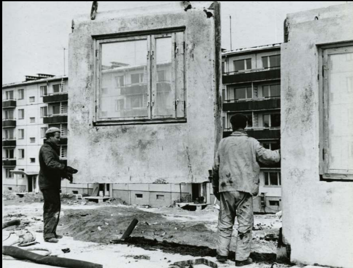
Mustamäe housing district. Window panel. Architects Voldemar Toppel, Toivo Kallas, Lidia Pettai. 1962.
