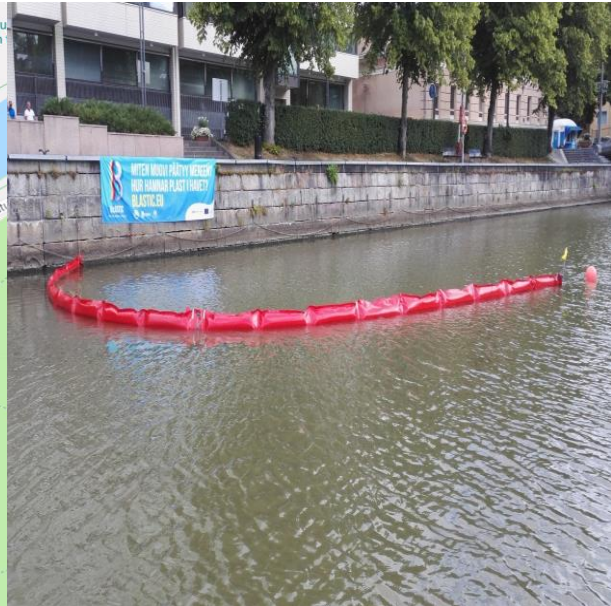
Figure 33. Downstream boom deployed in Aurajoki. Photo: Pekka Kotilainen.
