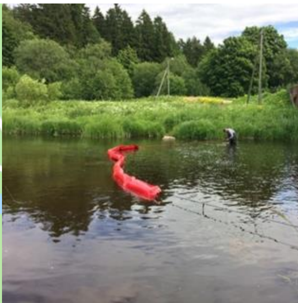
Figure 21. Installing of the boom set at Pirita Site 1.
