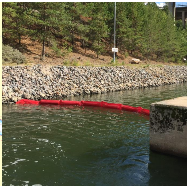
Figure 11. Boom 3 deployed at Södertälje channel bridge.
