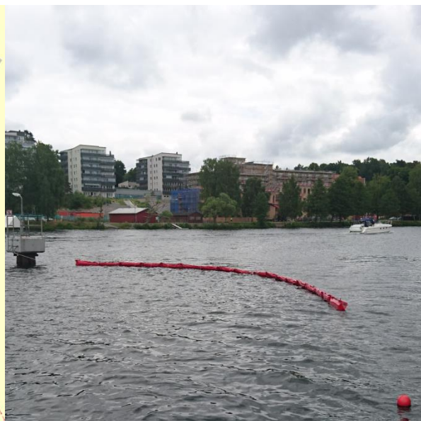
Figure 9. Boom 2 deployed at Södertälje channel inlet.
