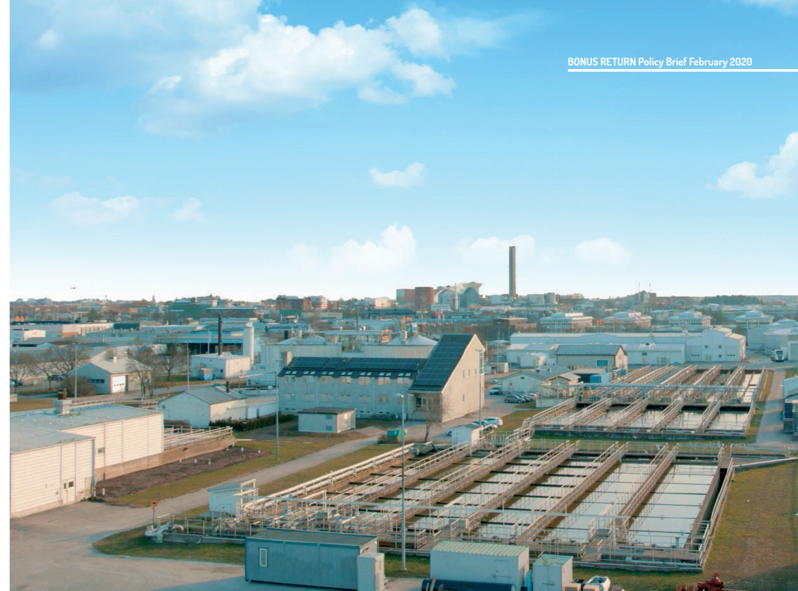
Uppsala wastewater treatment plant. Image: SEI
