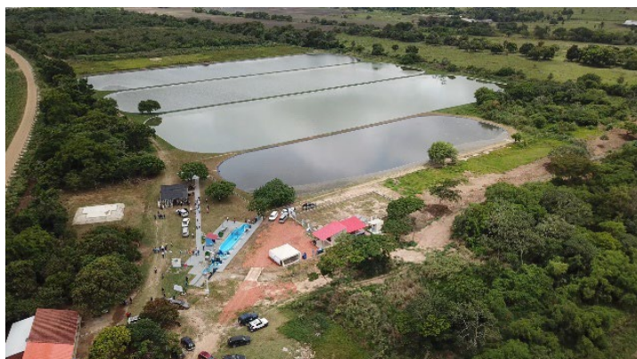
WSP in Montero (Source: Aguatuaya)
