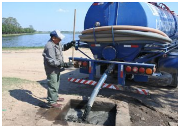
Septic tank, sludge collection and treatment at WWTP in Montero (Source: Gustavo Heredia)
