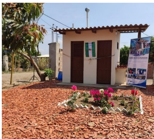
Dry, urine-diverting toilet and greywater garden in Montero (Source: UNICEF Bolivia)
