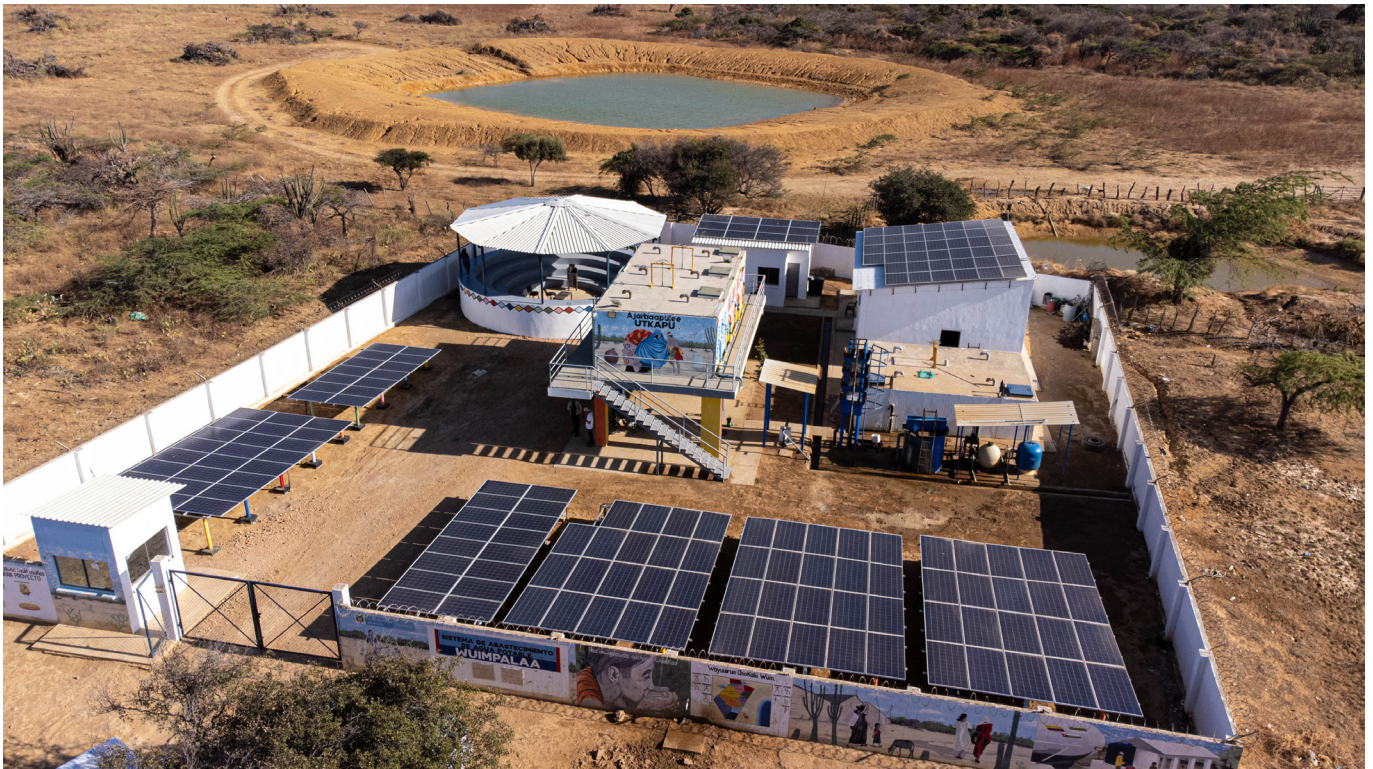
Wimpalaa microaqueduct in the Municipality of Maicao, La Guajira, associated benefit to the Windpeshi wind farm © EDUAR MONSALVE / SEI
