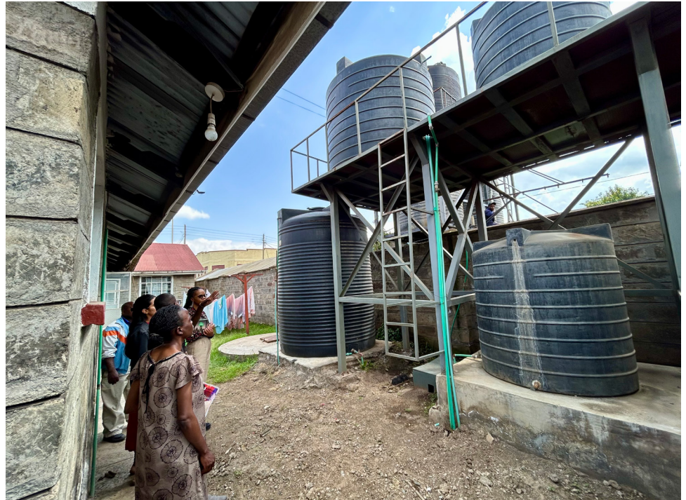
Figure 4. Water tanks in a public hospital in Nakuru being filled by pumping water from their own borewells, similar to the case in a private hospital in Bangalore. Water authorities do not charge for water drawn from private borewells.
