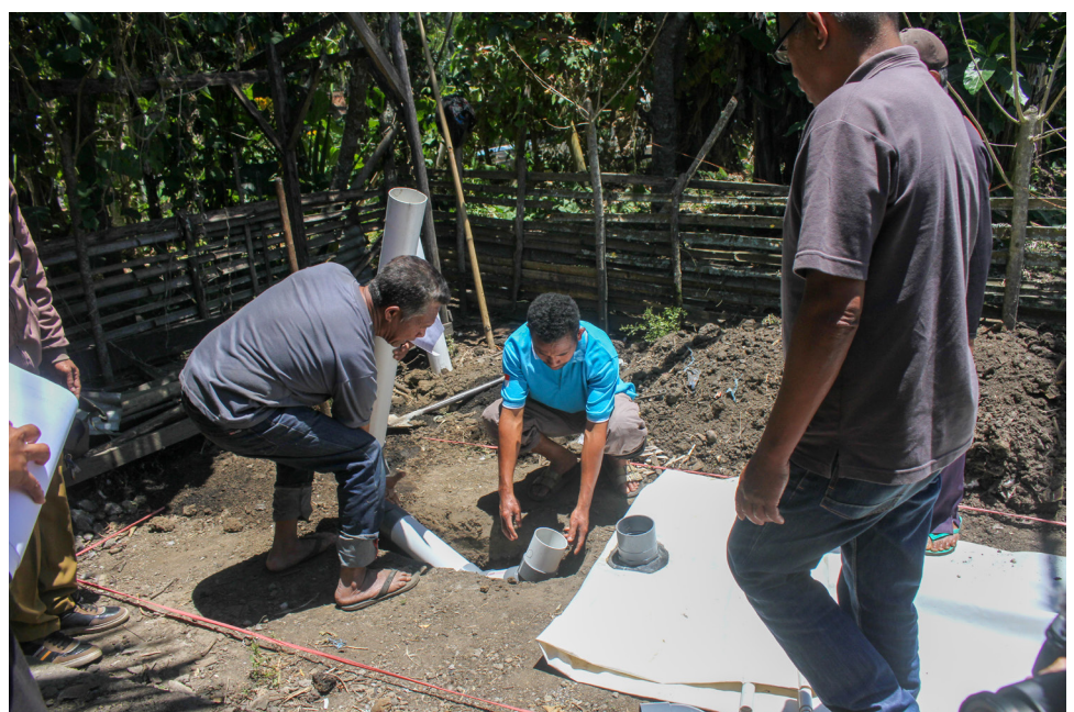
A biogas digester is being assembled and installed on a farm in Bajawa, Flores. September 2023. Photo credit: Cynthia Crouse
