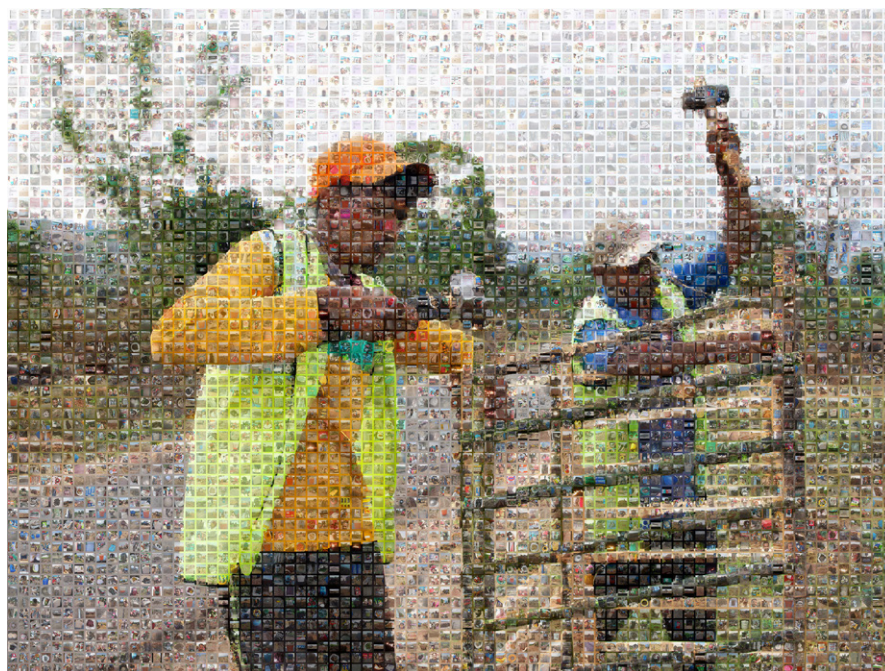
Workers install a tree guard for the 14 Trees Foundation, a locally led adaptation initiative. The picture is a mosaic of hundreds of photographs of on-ground economic transactions – “every gas cylinder bought, every wage paid, every tree guard installed” – created from a system in which every expense is logged with a photograph attached. As 14 Trees describes it, the image is “quite literally, the spend on the ground rendered visible”. Photo: 14 Trees Foundation, Vetale, Khed taluka, Pune district, Maharashtra, India
